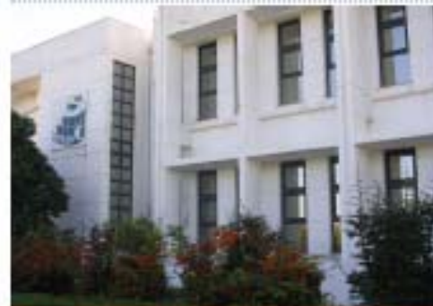
STEP-C's main building - the focus for the promotion of innovation in Heraklion, Crete.
